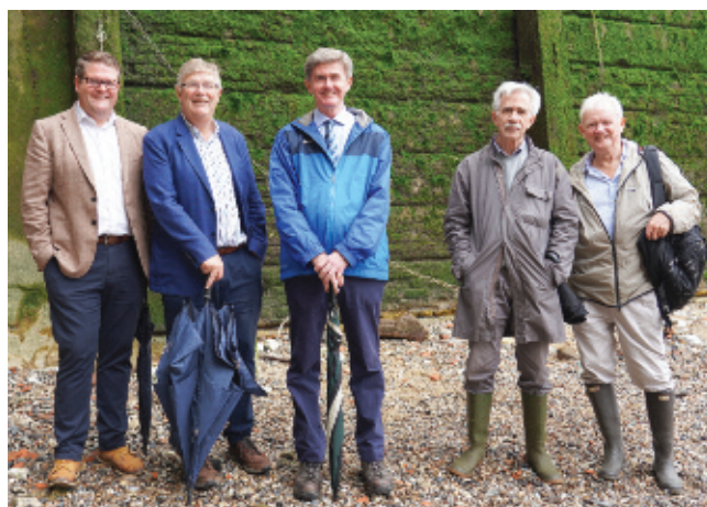
An intrepid band in their boots following their inspection of hitherto unseen exterior masonry faults which have led to water ingress at cellar level at Glaziers Hall.
